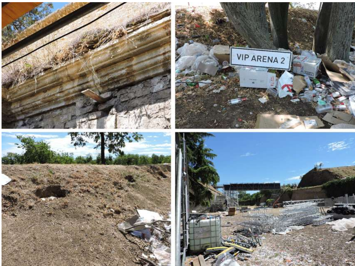
Fig. 3.6.1. Some deterioration post-Exit Festival Upper-left: Structural damage to a gate to facilitate passage of an electrical cable. Upper-right: Uncollected garbage. Lower-left: Structural damage from digging holes in the Fortress, resulting in water ingress and potential collapse. Lower-right: General view of the structural stress created by the festival's equipment.
